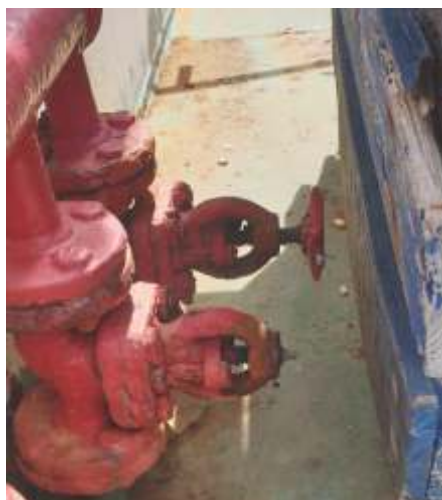
Damaged and blocked valves
