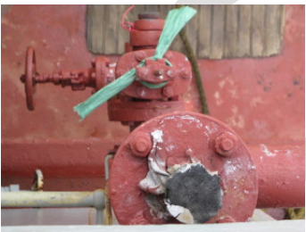
Pictures 4 - Fire Hydrant seized and hand-wheel missing
