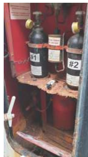
Co2 Locker corroded
