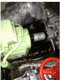
Picture 6 – Leaking Fuel Pump
