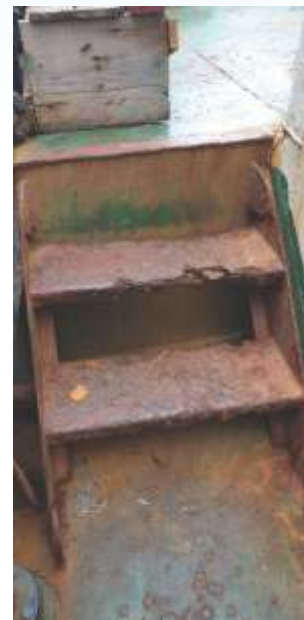
Corroded and blocked deck steps
