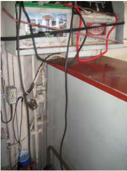
Picture 2 - Emergency lighting batteries discharged
