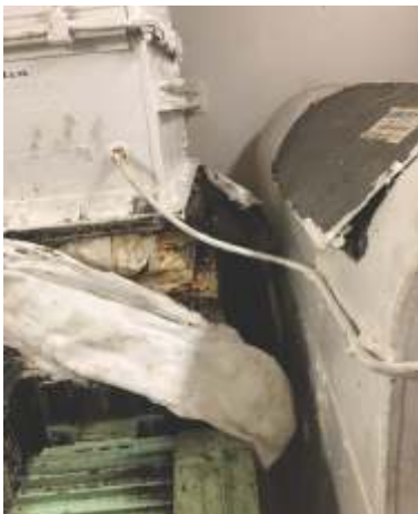
Galley fan with the cover lifted and insulation not in place
