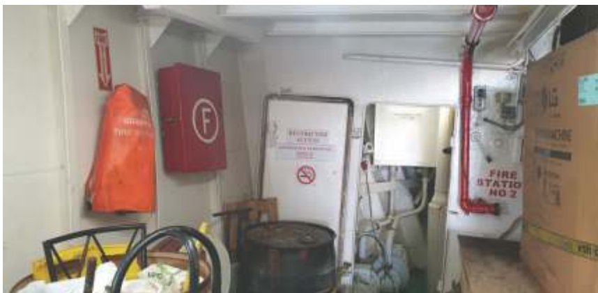
Fire fighting equipment blocked by pallets and boxes and not readily available for use
