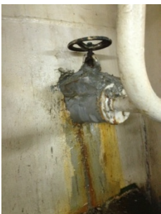
Picture 7 – Leaking Overboard Repaired With Cement
