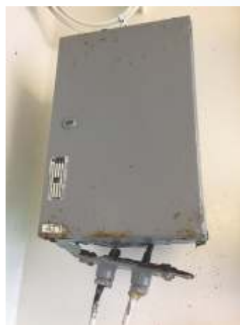
Electrical box off the bulkhead with the bottom falling out
