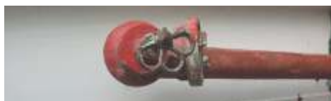
Damaged fire hydrant
